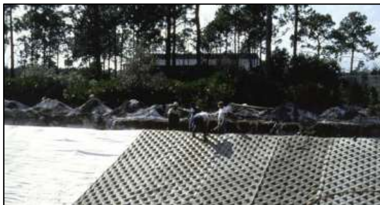
Fabric forms being filled with fine aggregate concrete.
